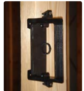
Backless brackets provide the minimum structure you'll need to attach a wall plate. If you're installing one to run speaker wires to your receiver, mount it at the same height as AC outlets for a clean, uniform look. If you're installing one for an IR sensor or volume control, mount it at the same height as light switches.
