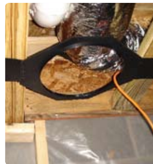
Hole-saving (or "rough-in") brackets tell the drywaller to cut a hole for the speaker (just like he/she would for electrical outlets and lighting fixtures). This makes your job much easier later on, since it takes the guesswork out of finding your speaker location and wire after the drywall's up.
